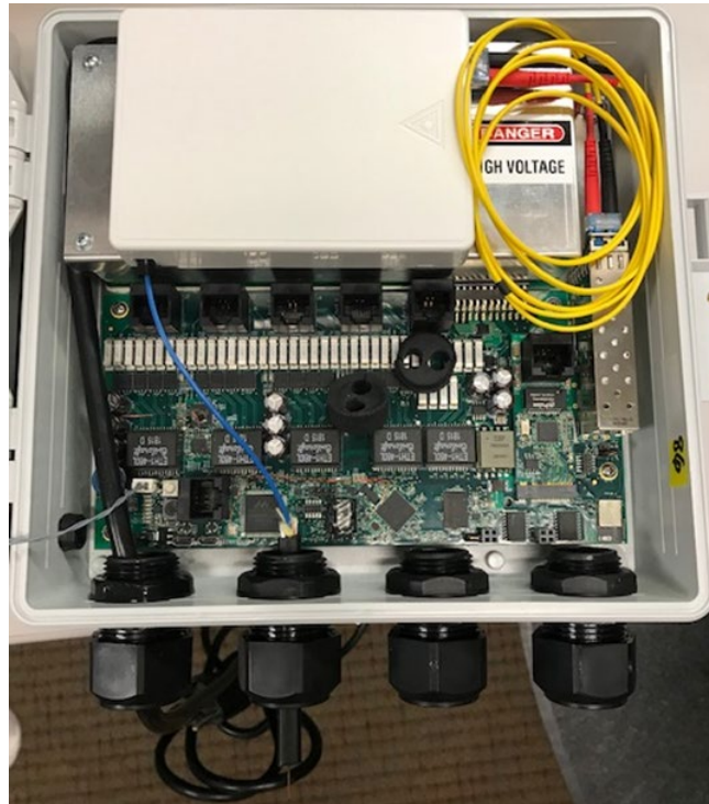
Fig. 7: Fiber Tray with Fiber Installed and Coiled with Lid On
